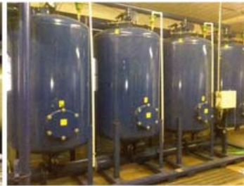
Water Plant Filters (during plant renovations) Iron Removal and Softening Plant
