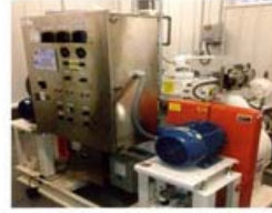
Lift Station with Gorman-Rupp Pumps
