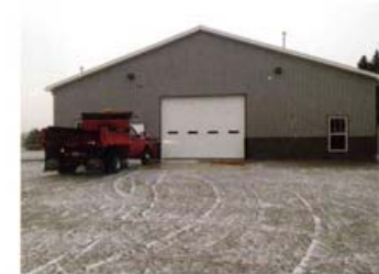
New DPW Building (From Back)
