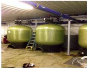
Water Plant Filters (during plant renovations)
