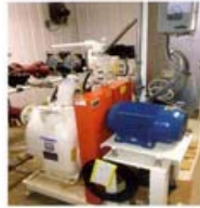
Lift Station with Gorman-Rupp Pumps
